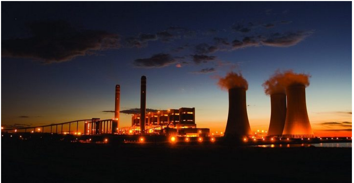
Pictured: Mabuja Power Station, Mpumalanga
